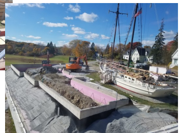
Getting ready to pour the slab under Schooner Gem's watchful eye.
